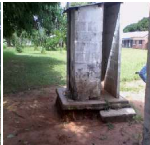
FIGURE 7: Latrine with clean floor and walls
