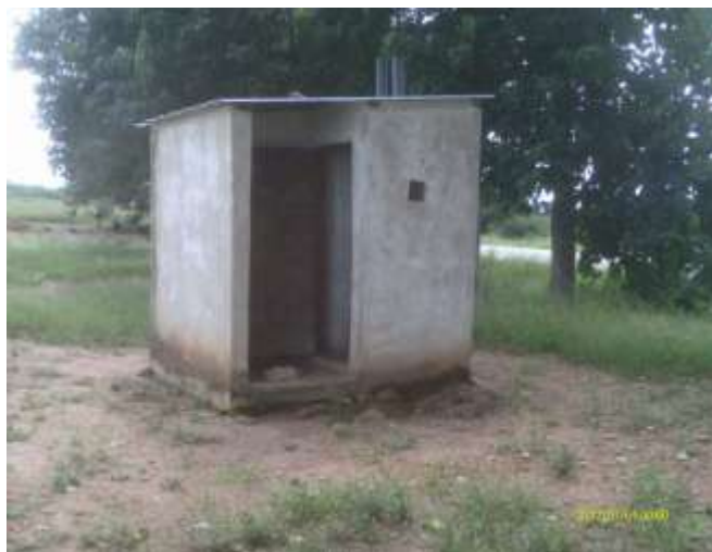
FIGURE 6: Latrine with a door
