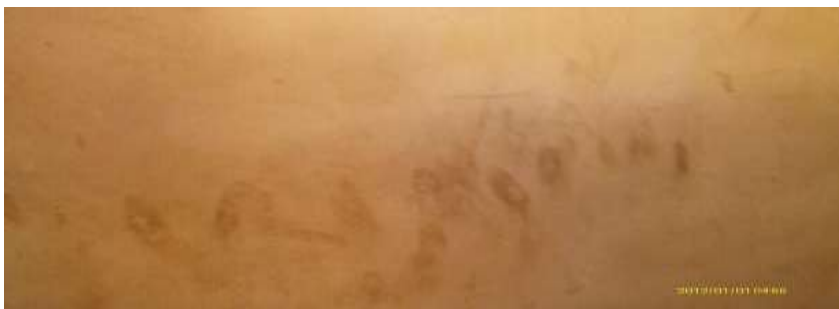
FIGURE 12: Picture of a latrine with fecal matter on the walls
