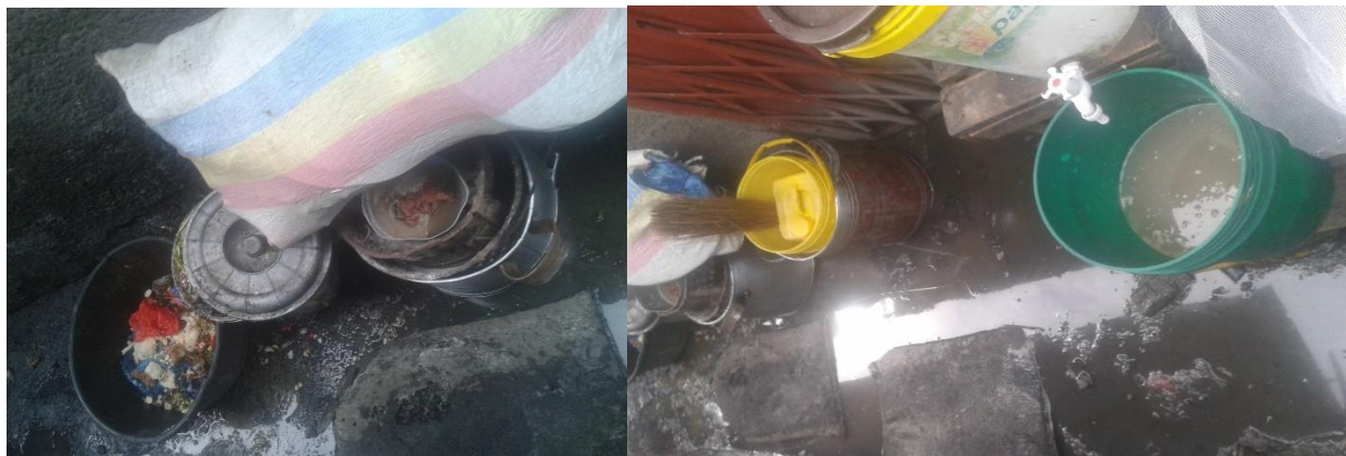
Figure 4: poorly drained wash-up area also used as storage for solid waste and utensil and is also a serving area
