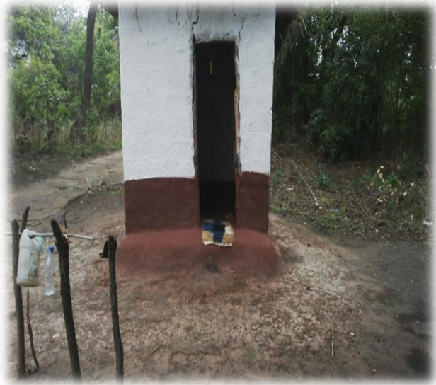
pit-latrine and tippy tap provide with soap in a small bottle at Ulu villages
