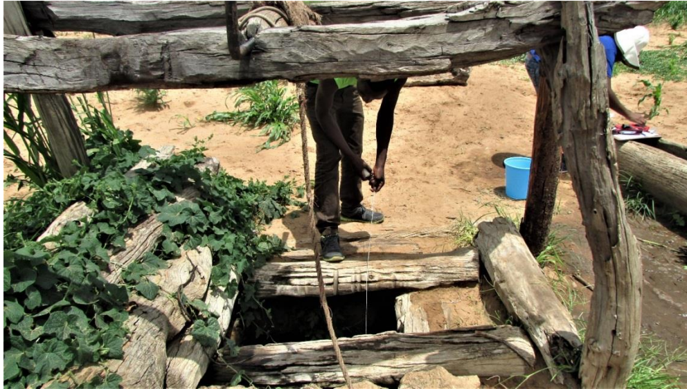
Figure 3.3: An illustrative diagram of the deep hand-dug wells found in the Omusati region of the Cuvelai Etosha Basin in which animals do not have access to the water.
