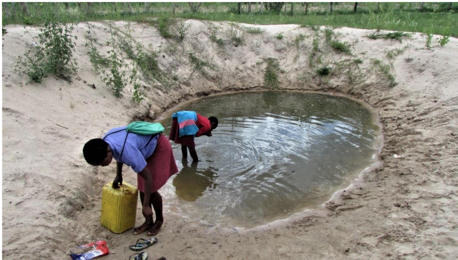
Figure 3.1: An illustrative diagram of the shallow hand-dug wells found in the Ohangwena region of the Cuvelai Etosha Basin in which animals have access to the water.
