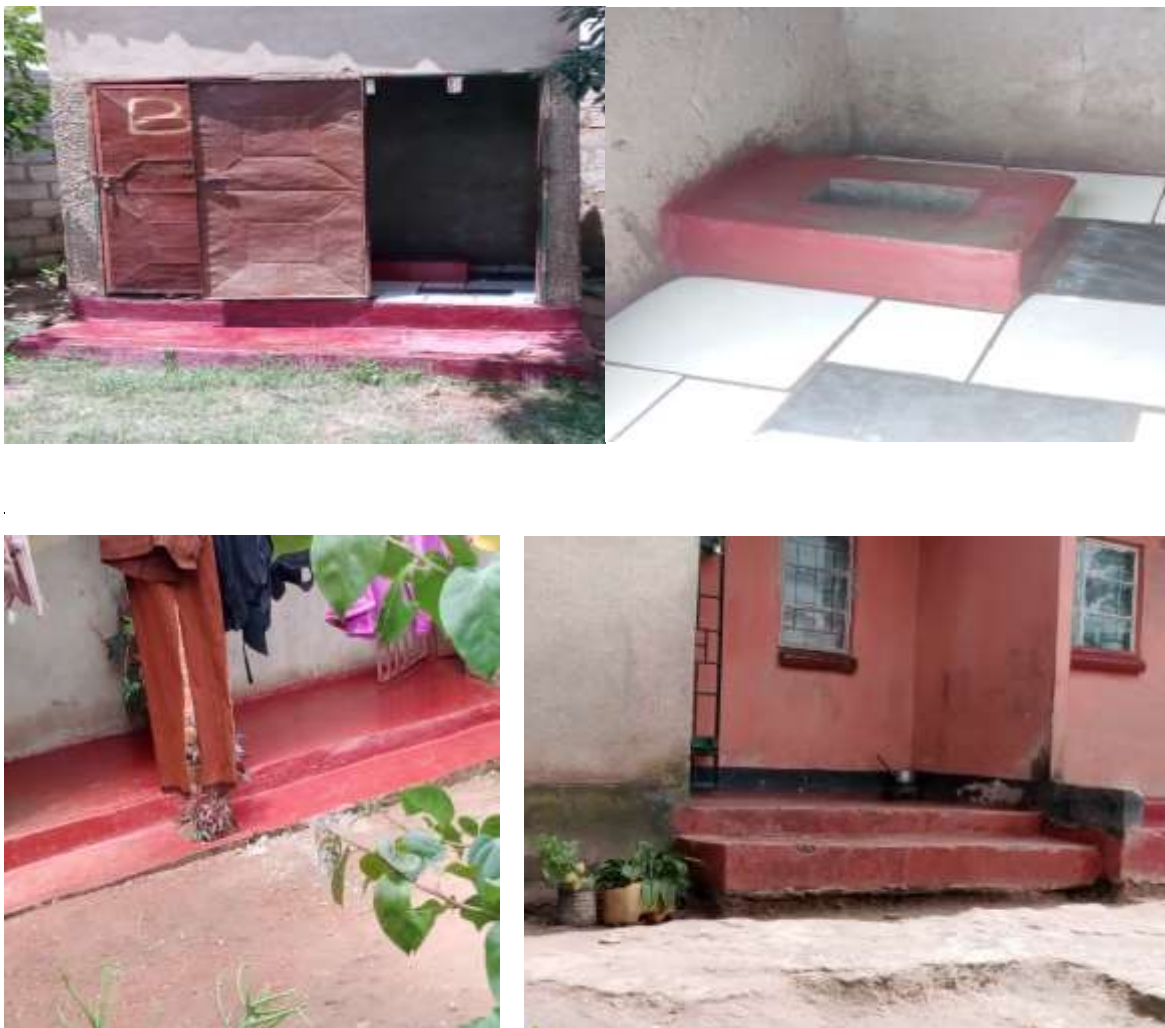
Picture 5: Clean pit latrine and swept surroundings.
