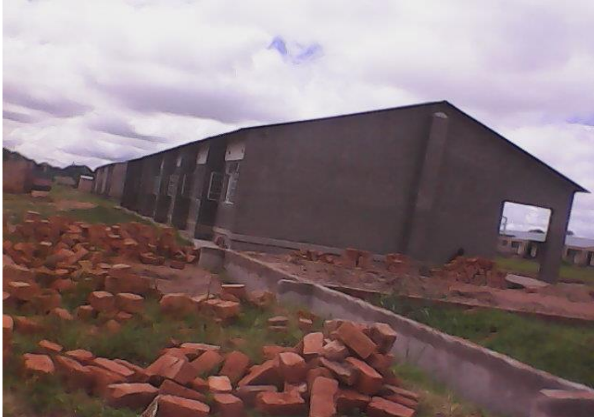
Figure 4.4: School B's PE classroom under construction
