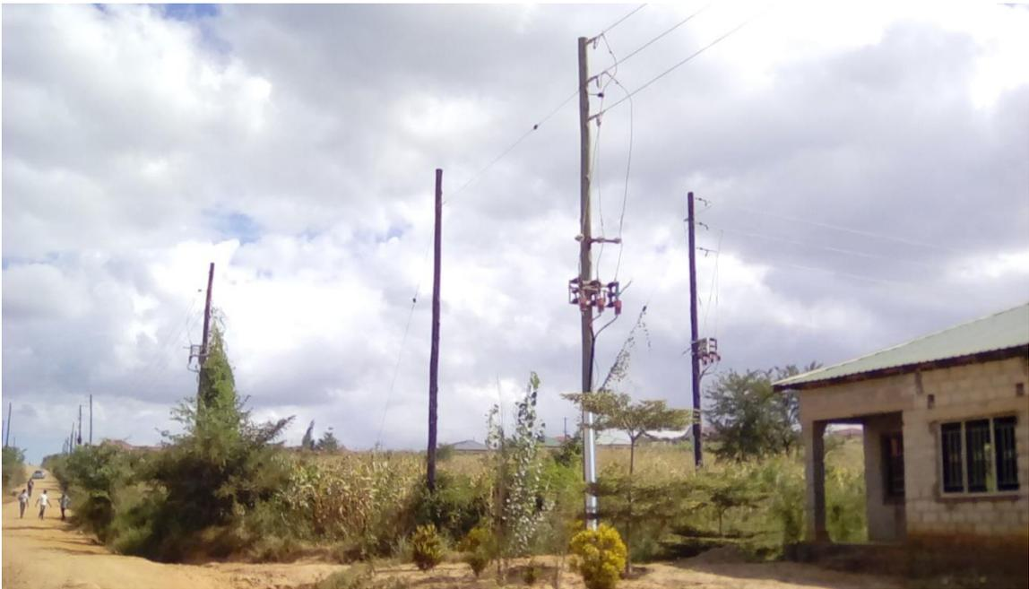
**Figure 3:** 11kV lines take off points feeding Kwamwena area
