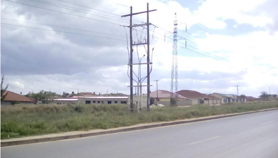
**Figure 2:** 33kV distribution line tapping point to Kwamwena substation
