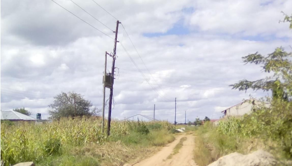
**Figure 4:** 100kVA 11/0.4kV transformer feeding households
