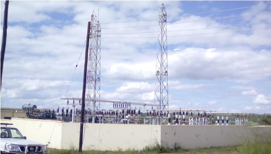
**Figure 1:** 31.5MVA 33/11kV Kwamwena substation
