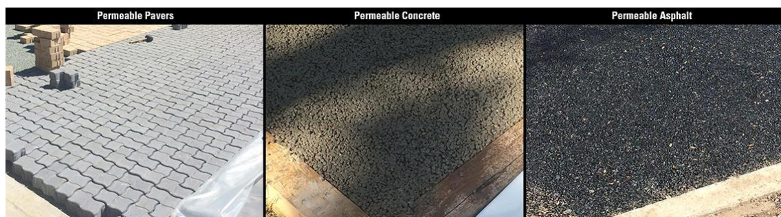
Figure 1: Types of pervious pavement systems. (Selbig and Buer, 2018).
