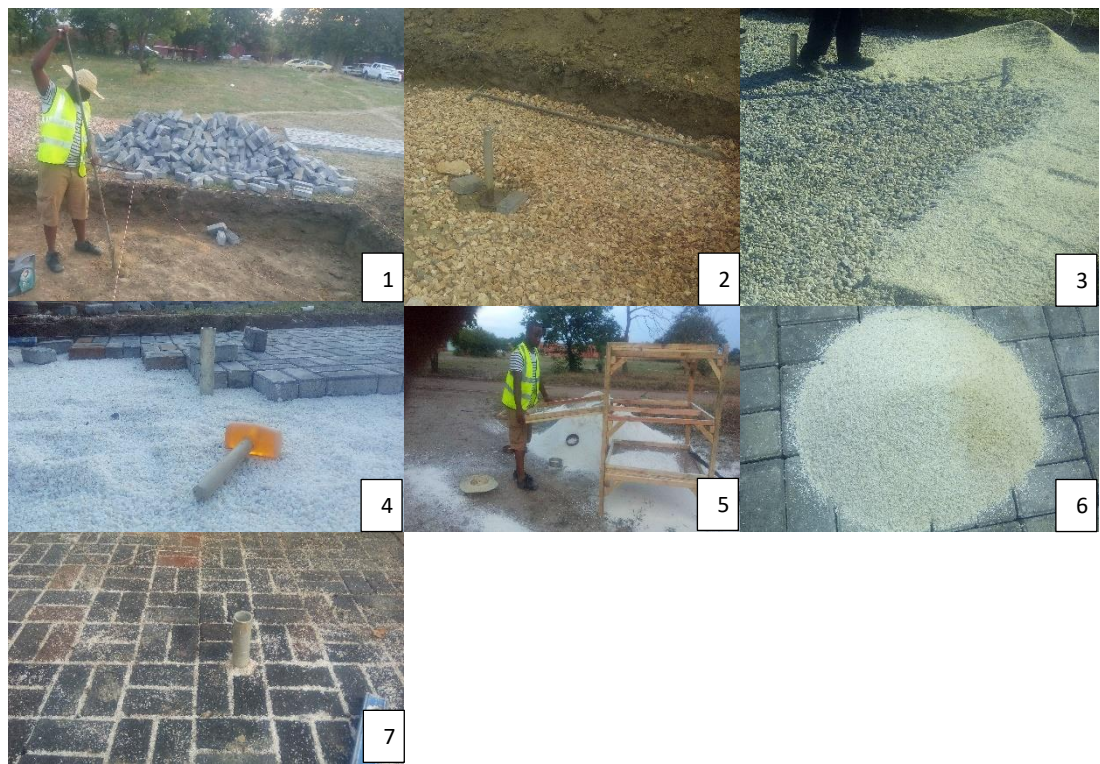
Figure 7: Installation of pavers after spreading the bedding layer.
