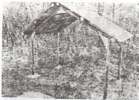
Figure 3: Use of nailed flitch plate BRE method in portal frames.
