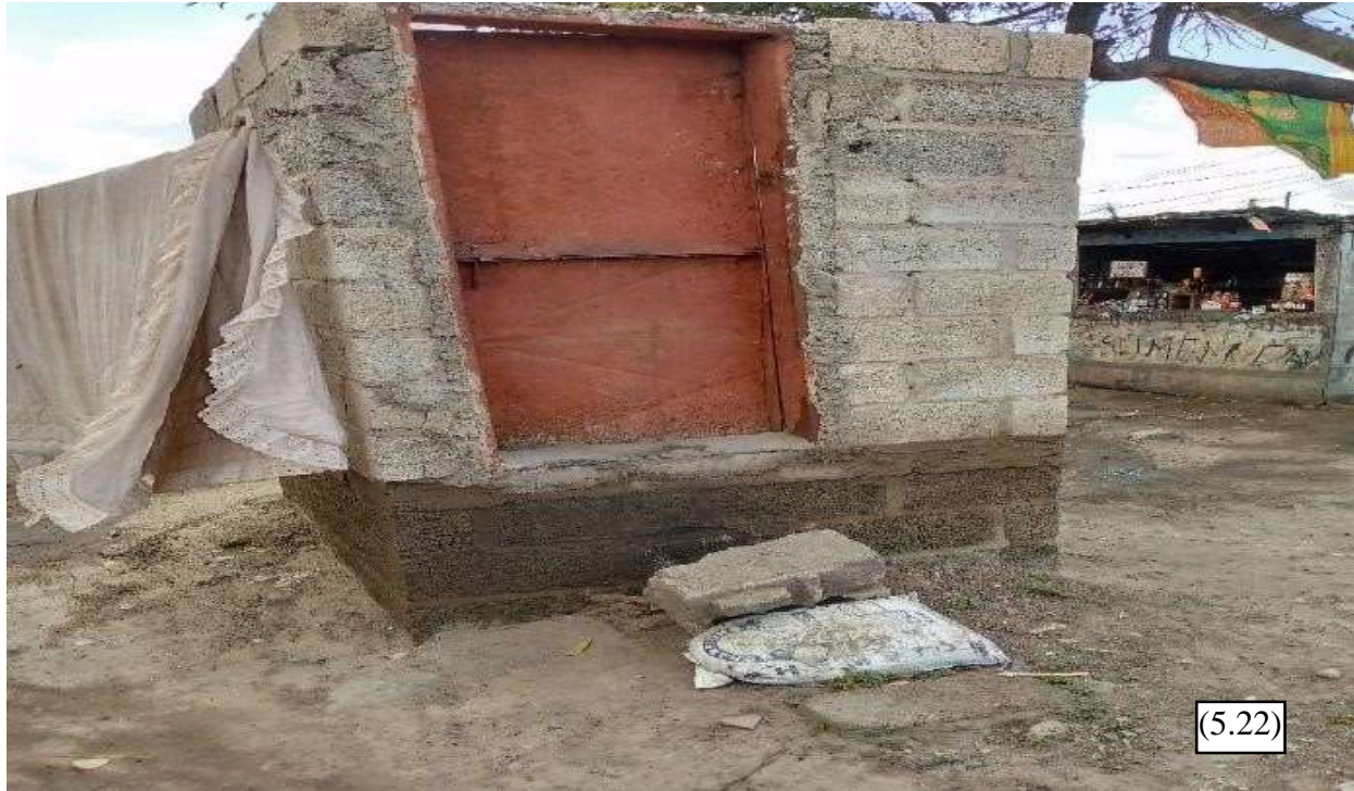
Figure 5.22: Pit latrine constructed at a higher elevation in Kuku to prevent floods in the latrine. This indicates the severity of flooding experienced.
