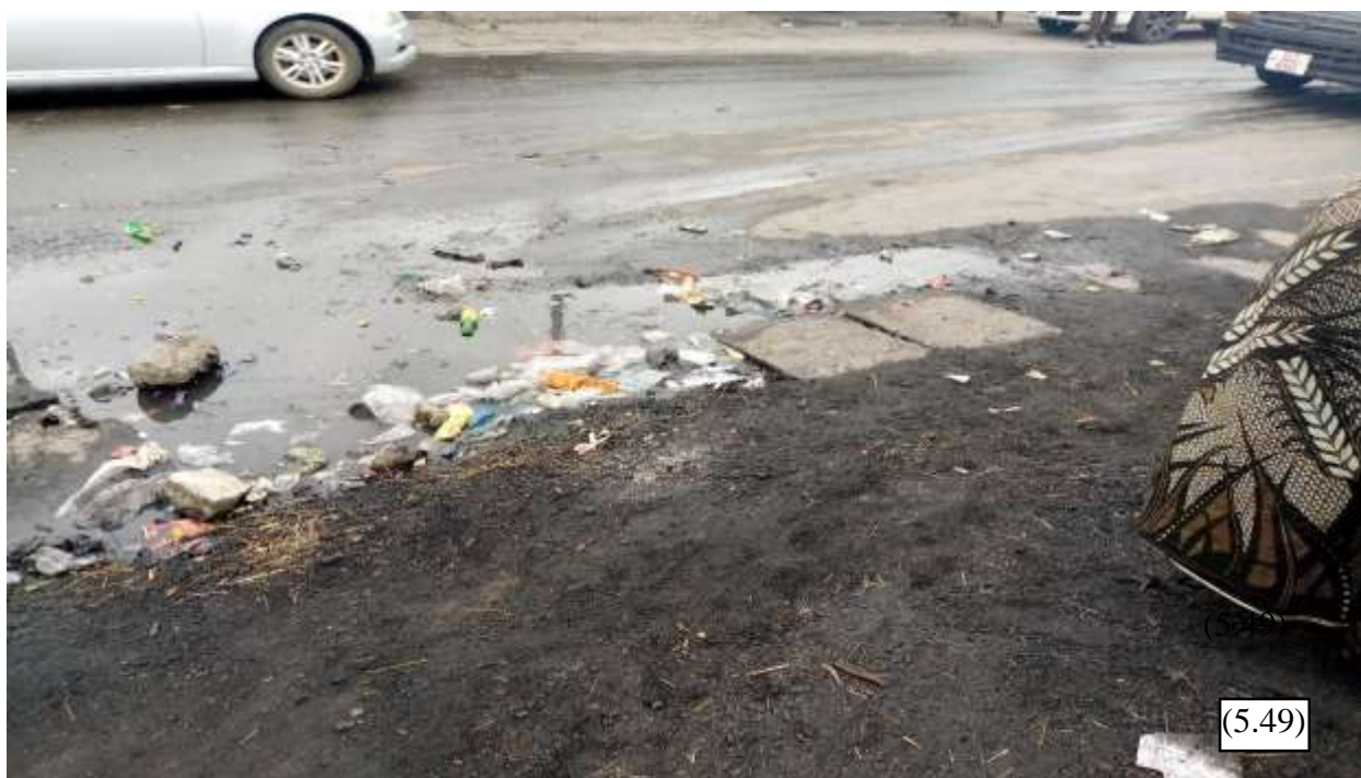
Figure 5.49: Blocked shallow drainage turned into a dumping site along kuku road prior the rain season
