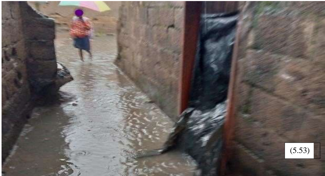
Figure 5.53: Vertically elongated black plastic strategically is over the outside wooden door to allow rainwater pour on it and flow directly outside without flowing into the house Source: Field data (2023)
