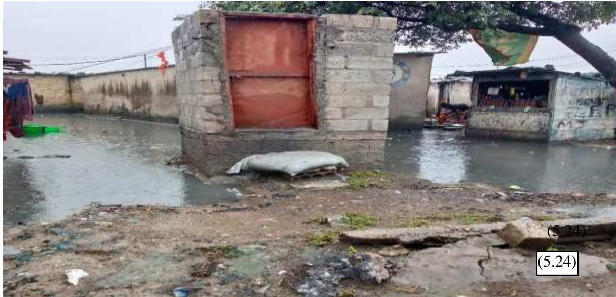
Figure 5.24: Same Pit latrine constructed at a higher elevation to prevent flooding in Kuku residential area during the rainy season as shown prior to the rainy season in figure (5.22) Source: Field data (2023)
