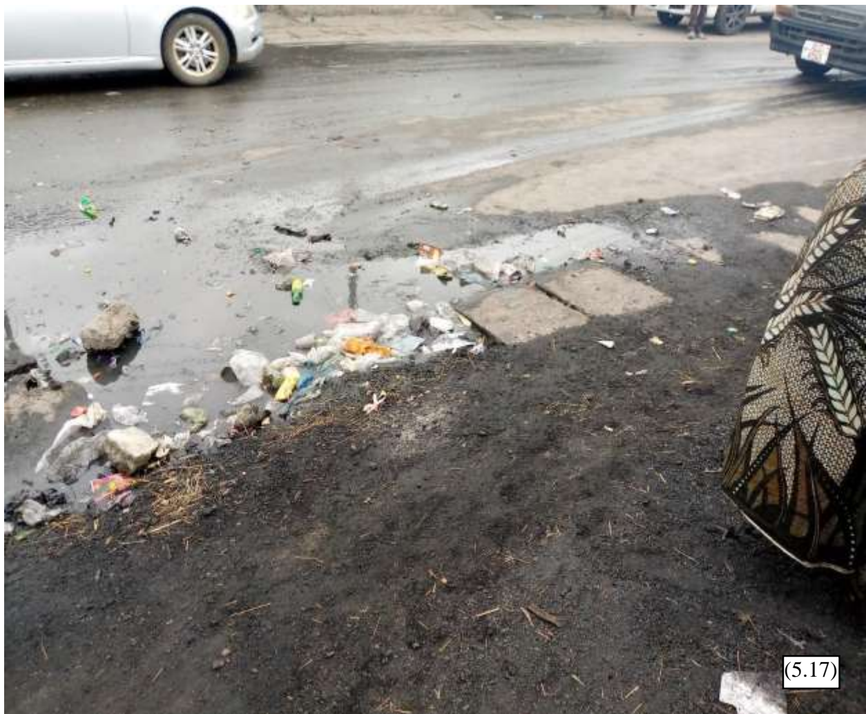
Figure 5.17: Blocked drainage turned into a dumping site along kuku road Source: Field data (2022)
