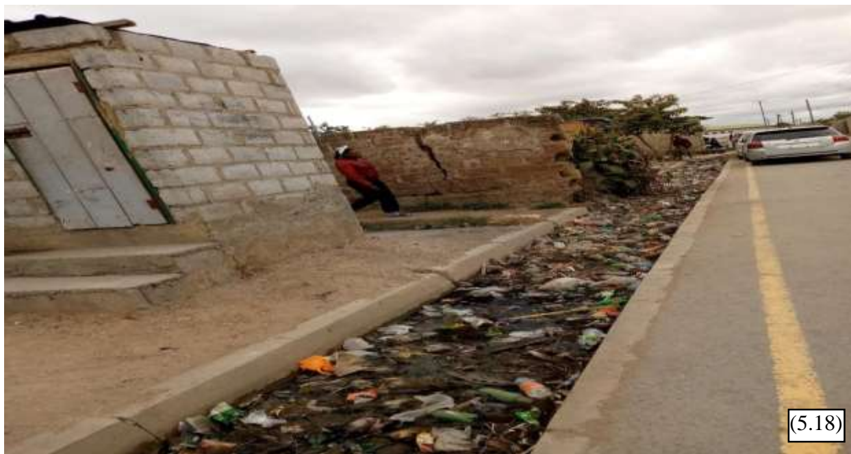
Figure 5.18: Drainage along the road filled with garbage and stagnant water in Kuku Residential area.
