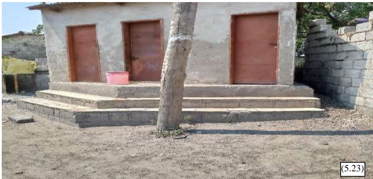
Figure 5.23: Pit latrines constructed at a higher elevation in Kuku to prevent floods in the latrine. This indicates the severity of flooding experienced.
