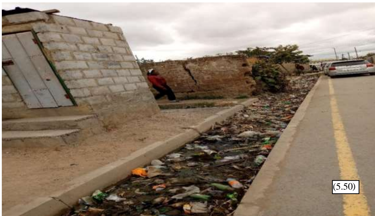
Figure 5.50: A swallow drainage along the road filled with garbage and stagnant water in Kuku residential area before the rainy season
