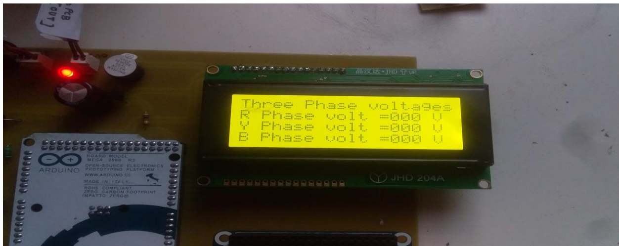
Figure 4.8 Voltage Values of the Three Phases Displayed Showing Zero Voltage
