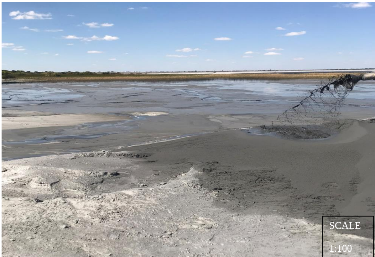
Figure 2.5: Site pictures from the Mopani TD15A tailings dump showing fine grained material and tree cover on the slopes of the dump.
