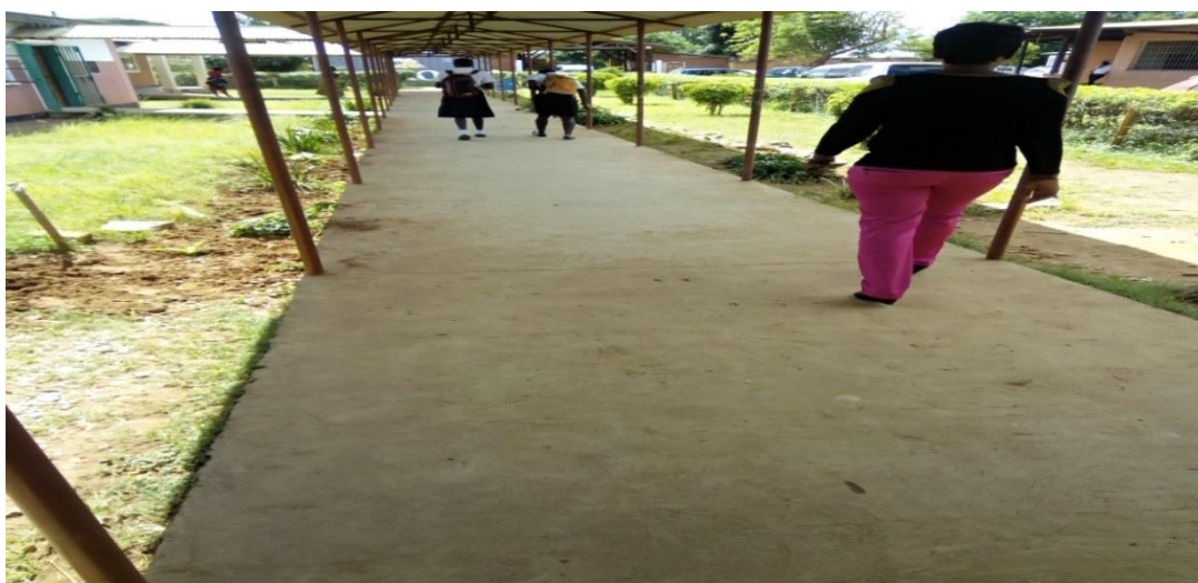
Figure 14: An accessible corridor at Don School ( Source: Field data, 2018 )
