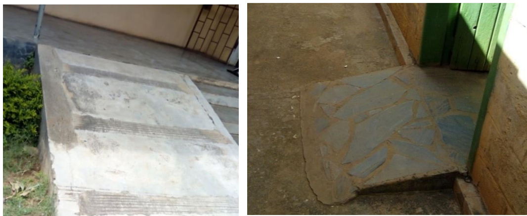
Figure 17: Ramps at Venus (left) and Don schools (right) (Source: Field data, 2018)
