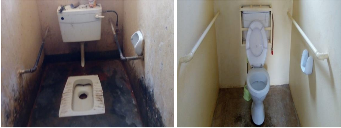
Figure 20: Toilets with grab bars at Dudu (left) and Don (right) ( Source: Field data, 2018 )
