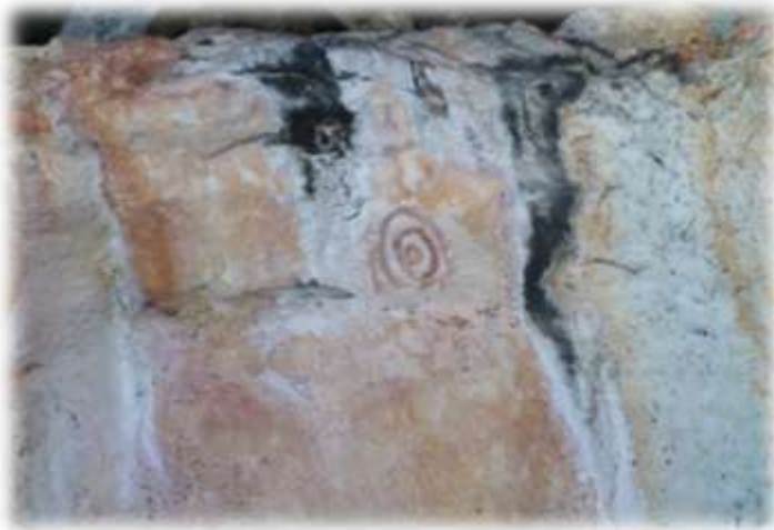
Figure 20: Deposition of insoluble salts, or minerals, over the walls at site KRS-3.
