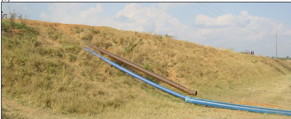
Figure 6: Photographs showing (a) excavated ditches in the upland areas of Chassa dambo and (b) the northern dam wall in Chassa dambo, October 2009. Source: Field data.
