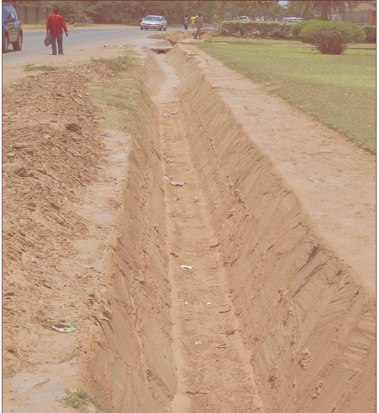
PHOTO 6: LCC at work! Removing soil from drainage along Kudu Road in Kabulonga Ward
