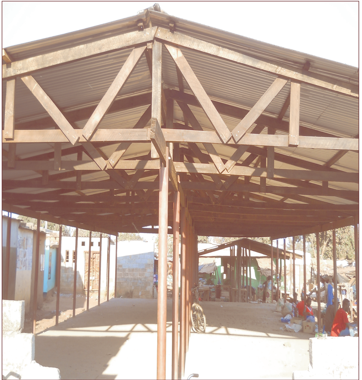
PHOTO 8: LCC at work! Construction of a Vegetable Shelter at Linda Market
