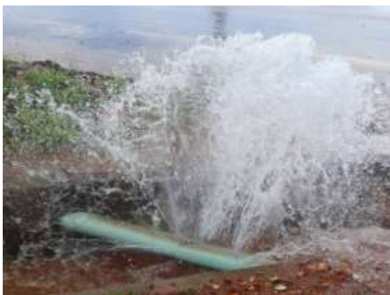
Figure 4.1: Burst PVC pipe
