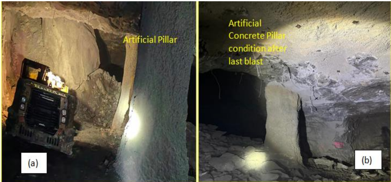
Figure 3.14: Condition of the artificial pillars during production loading from draw-points (a) and the condition of the artificial pillar after the last blast (b)
