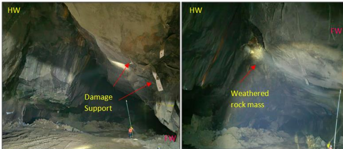
Figure 3.7: Status of the SA 1575 Stope before artificial pillars were installed
