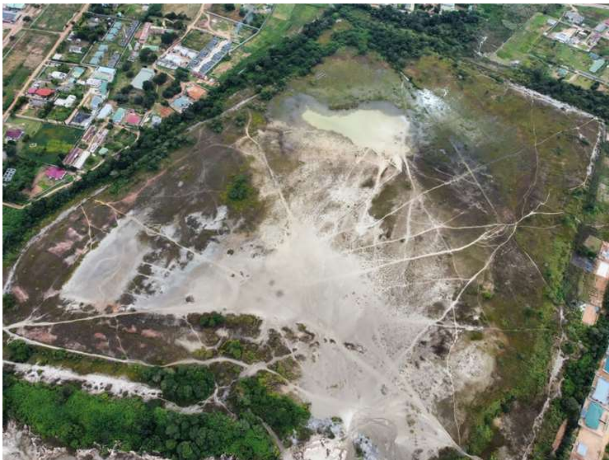
Figure 2b: Image captured by the Drone (DJI Mini 2) revealing TD27's vastness from an aerial perspective, Uchi Tailing Dump, Kitwe, Zambia
