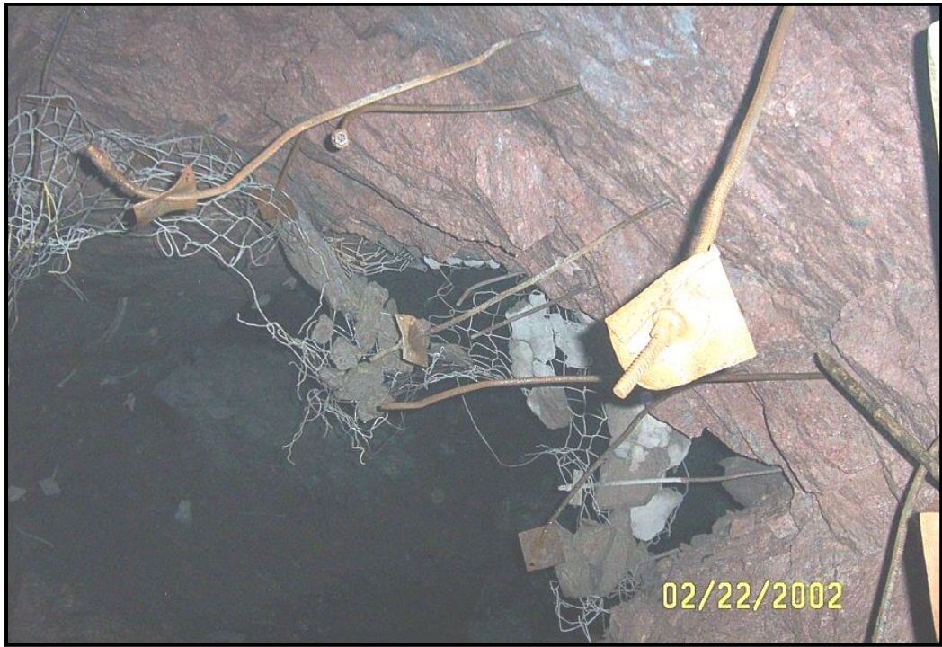
Figure 4:18: 2900L 570 mS Footwall Haulage rockburst event (Mutale, 2004)
