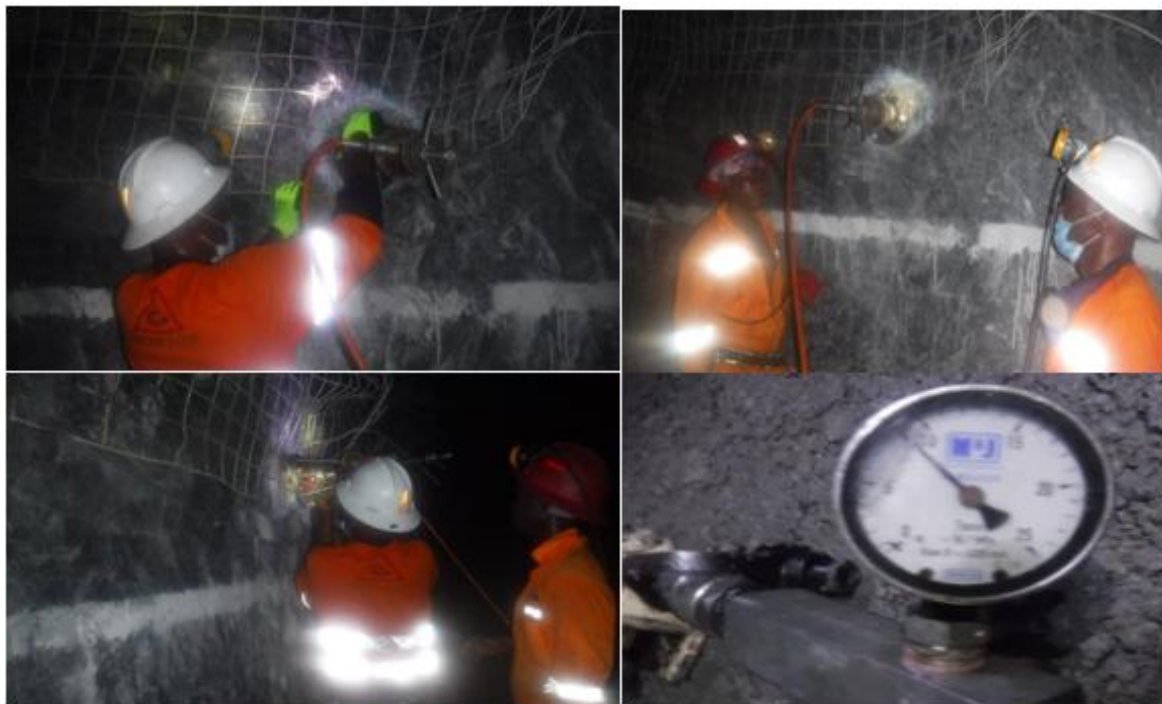
Figure 4.24: Group Four Minerals Ltd specialists mounting the Pull Test Rig
