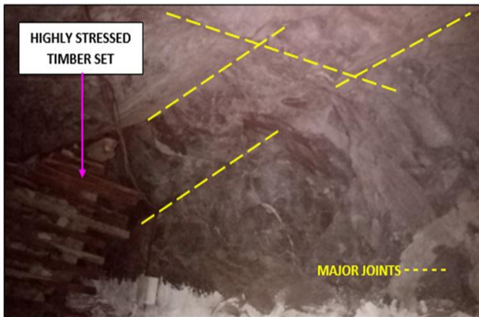
Figure 4.12: Timber pack under a jointed and stressed rock mass
