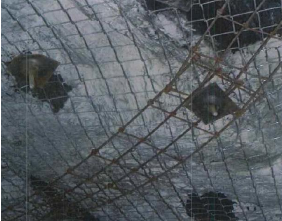
Good Rock Bolt support (100mm stick-out); 3240 LEVEL
