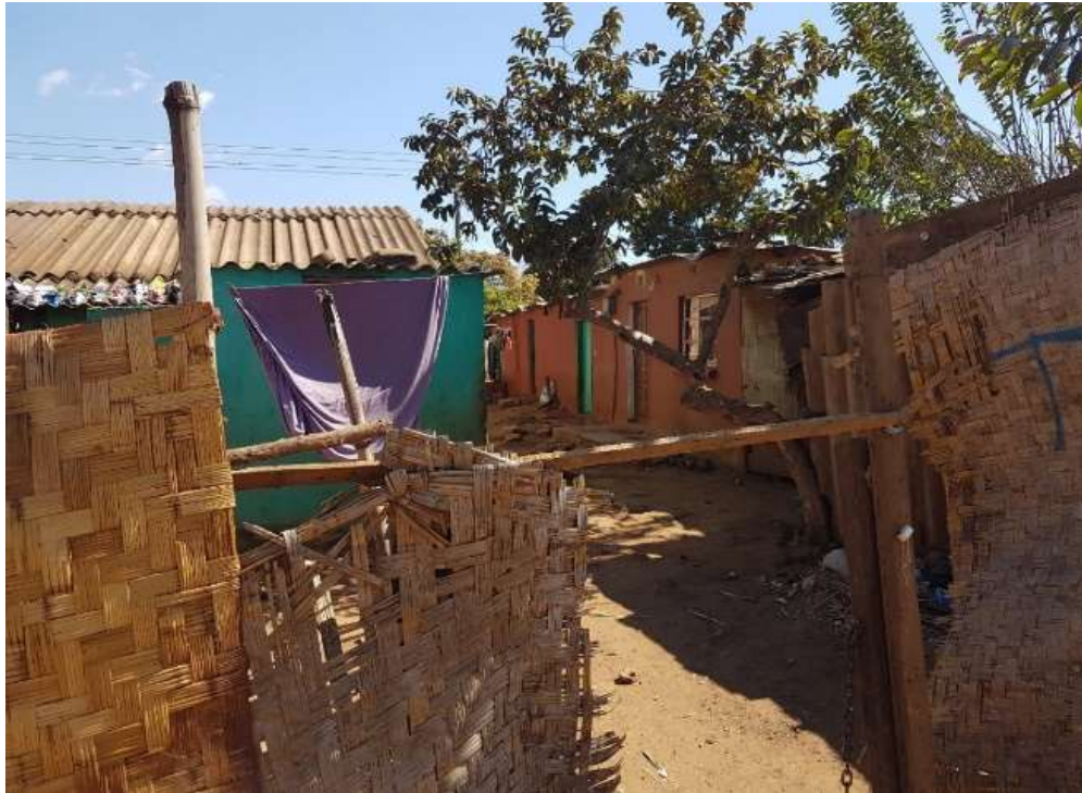
Plate 5. 5 Additional unit of three rental rooms
