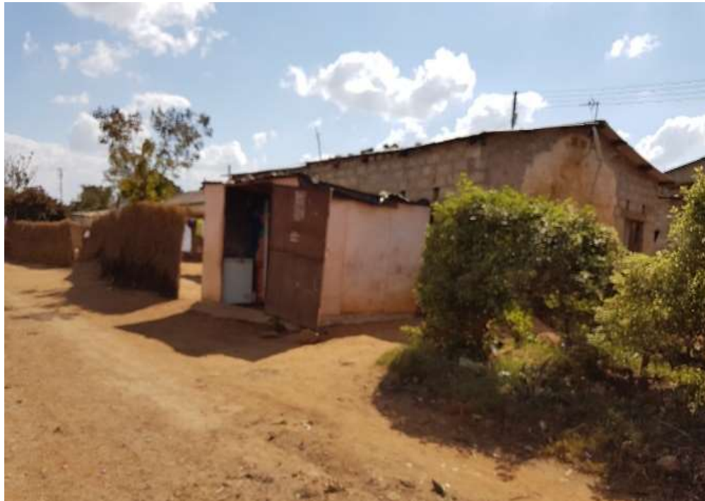
Plate 5. 6 Shop and extension to original house
