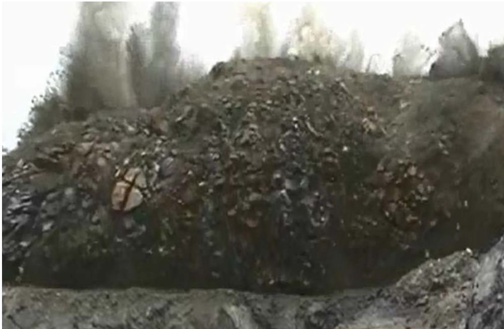
Figure 8: Bench blasting (MAXAM, 2010)
