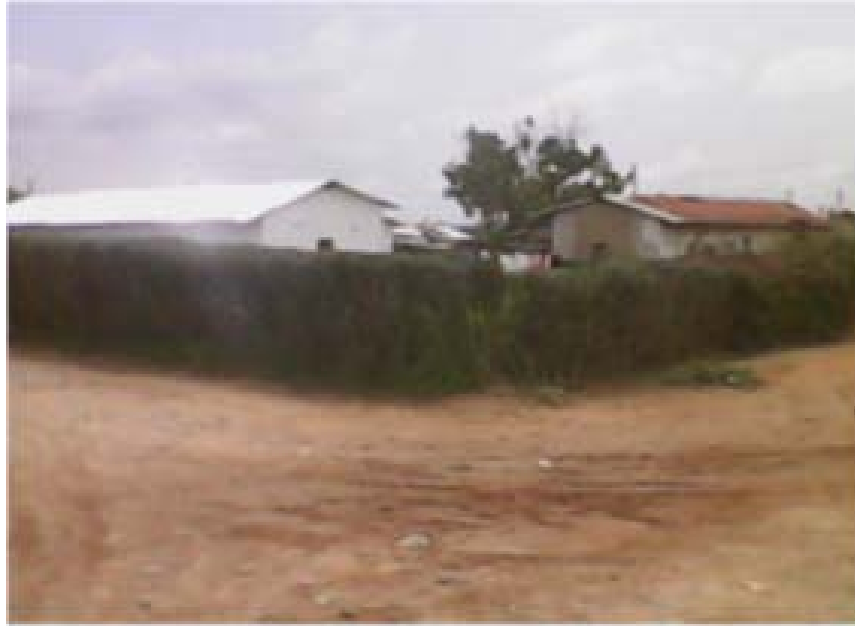
Figure 3: The condition of housing units in Wusakile close to the pit
