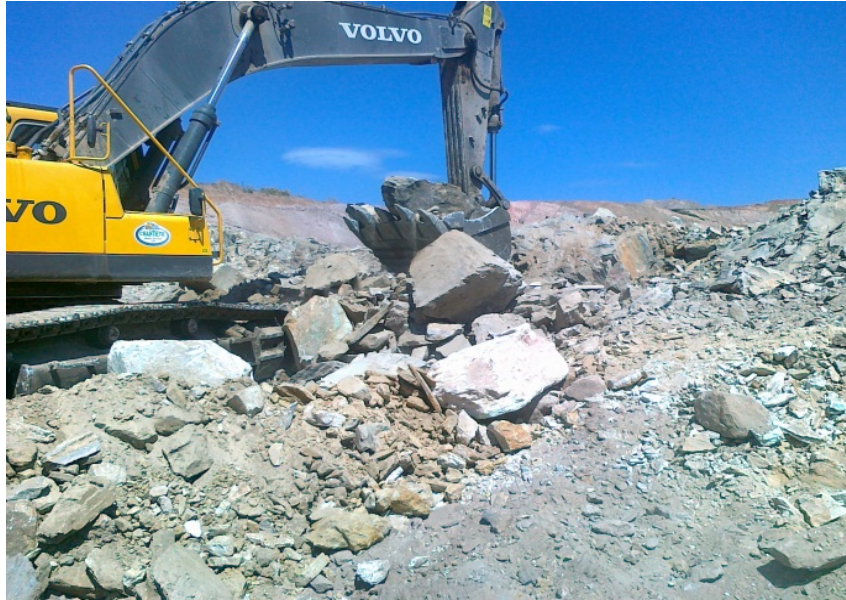
Figure 6: An excavator handling big boulders in the pit
