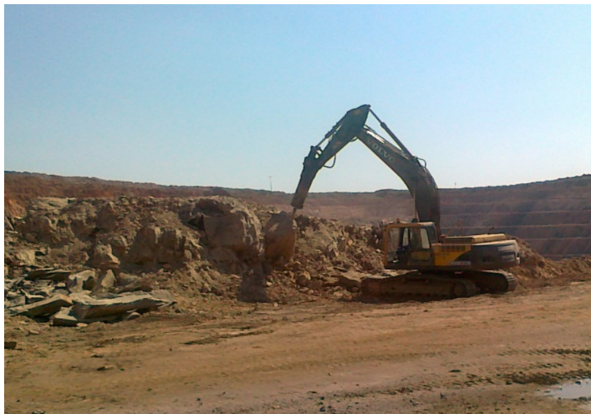
Figure 7: Rock breaker downsizing big unbroken rock at Area J
