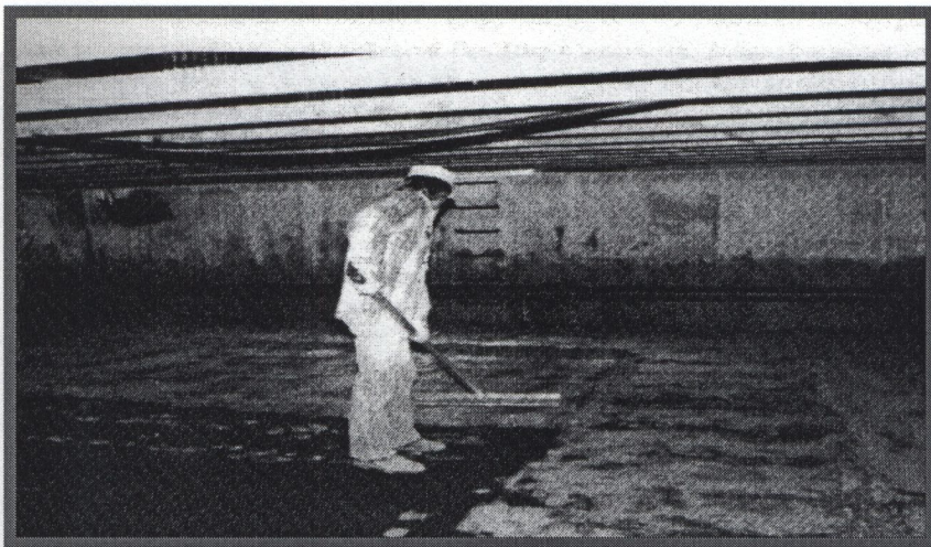
Figure 2.2-3: The scraping operation during cleaning of slow sand filters [ Source: Barret et al. , 1991]
