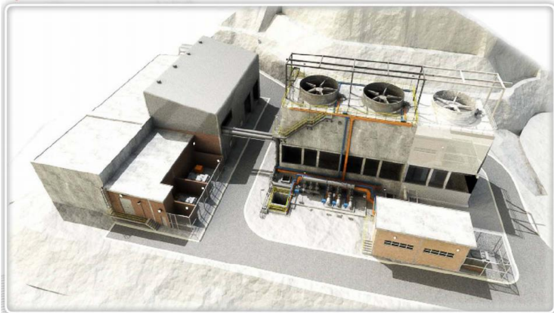
Figure 38: Surface refrigeration supplying cold water underground (Ramsden & Von Glehn, 2012)
