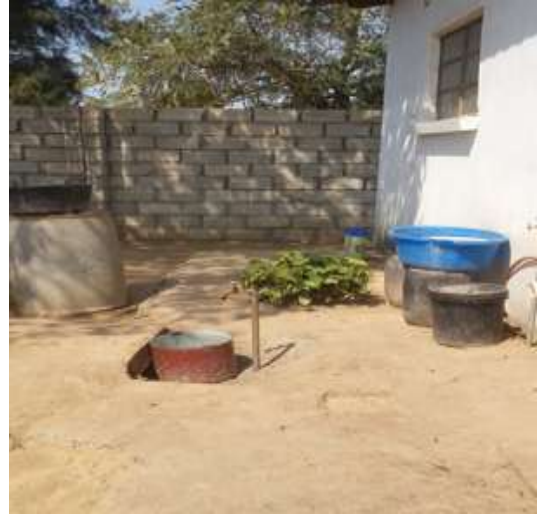
Figure 4: Piped water into yard in Chainda Shanty Compound, Lusaka, Zambia.
