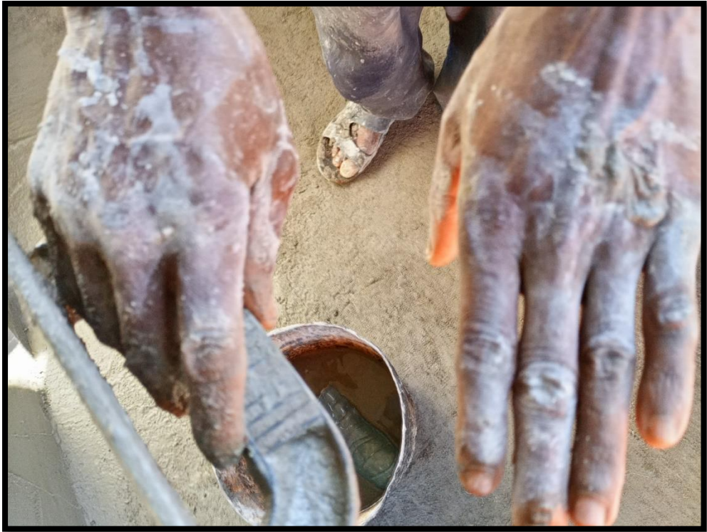
Figure 4.32: Picture showing exposure to wet concrete without PPE on a building project
