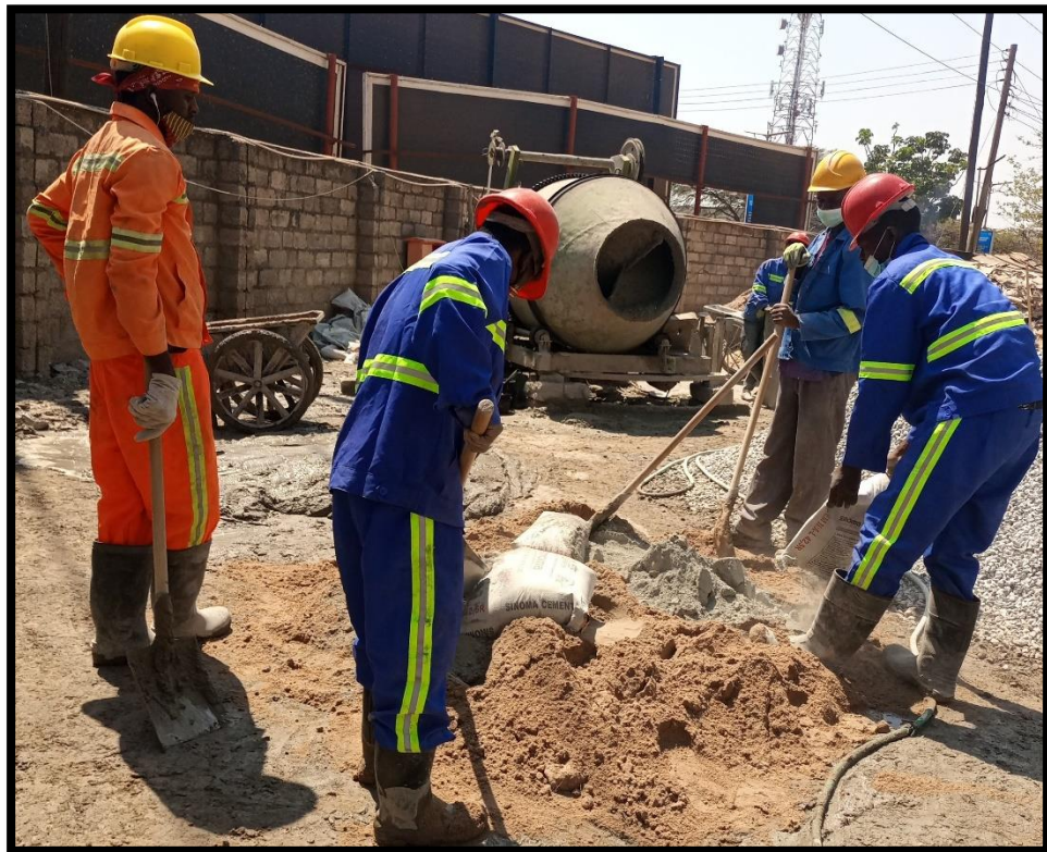
Figure 4.31: Picture showing some of the workers in gumboots
