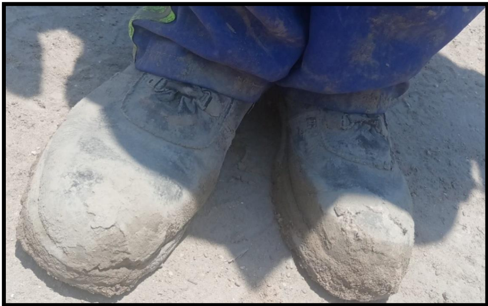
Figure 4.33: Picture showing wrong PPE for working with wet concrete
