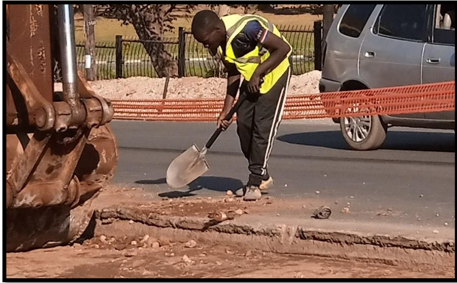
Figure 4.26: Picture showing dust control using water on the road project
