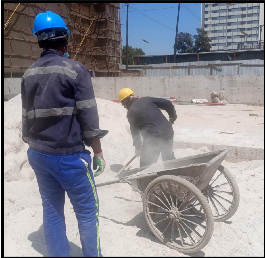
Figure 4.10: Picture showing workers loading quarry dust for batching
