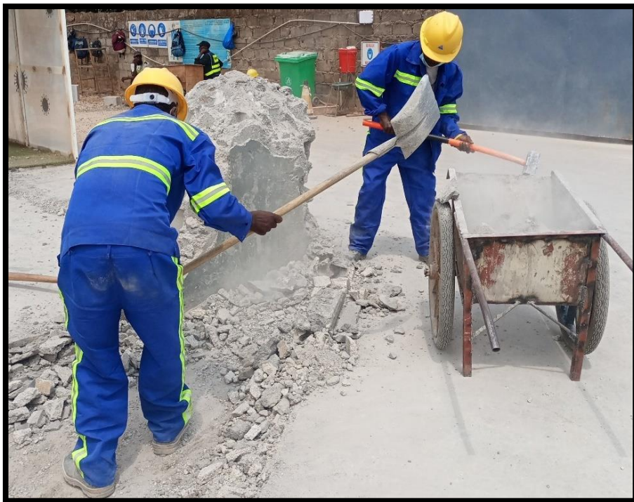
Figure 4.13: Picture showing dust exposure during demolition and loading of rubble
