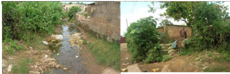
Figure 2-2: Housing with poor drains and covered with solid waste Source: Author, 2015
