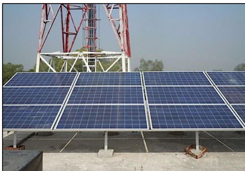
Figure 2-1: Escotel Solar Powered Mobile Telecommunication Tower
