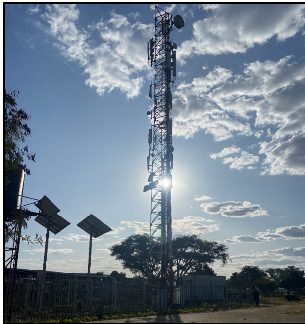
Figure 3-3: Telecommunication Towers built near municipal facilities
