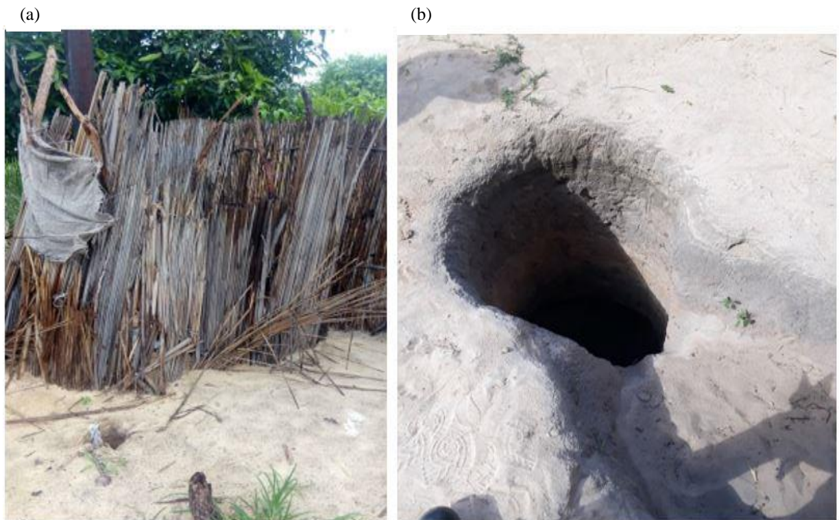
Figure 9: Pit latrine (a) within the radius 30m from a scoop hole (b) at Ngweshi Village (MW05) in Lukulu District, Western Province, Zambia
