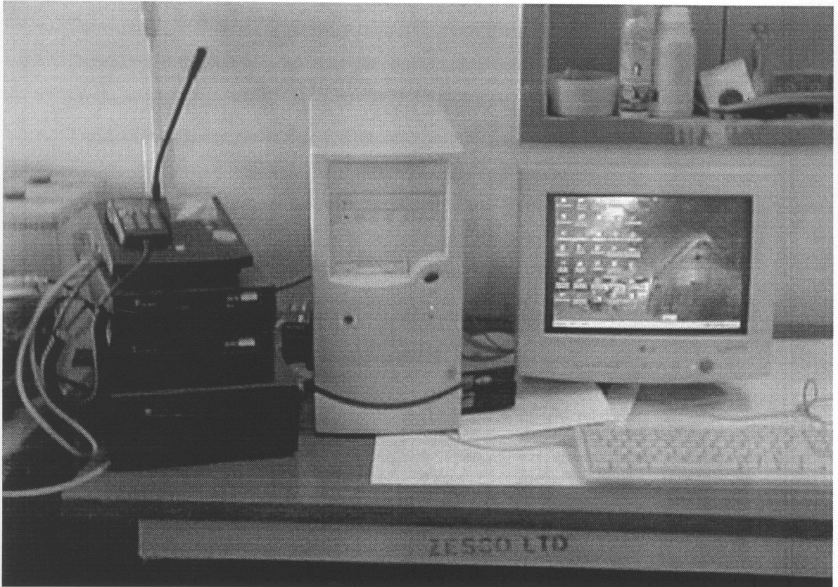
Figure1.1 Showing communication radio/modem interface to PC at Master station (ZESCO ltd)
