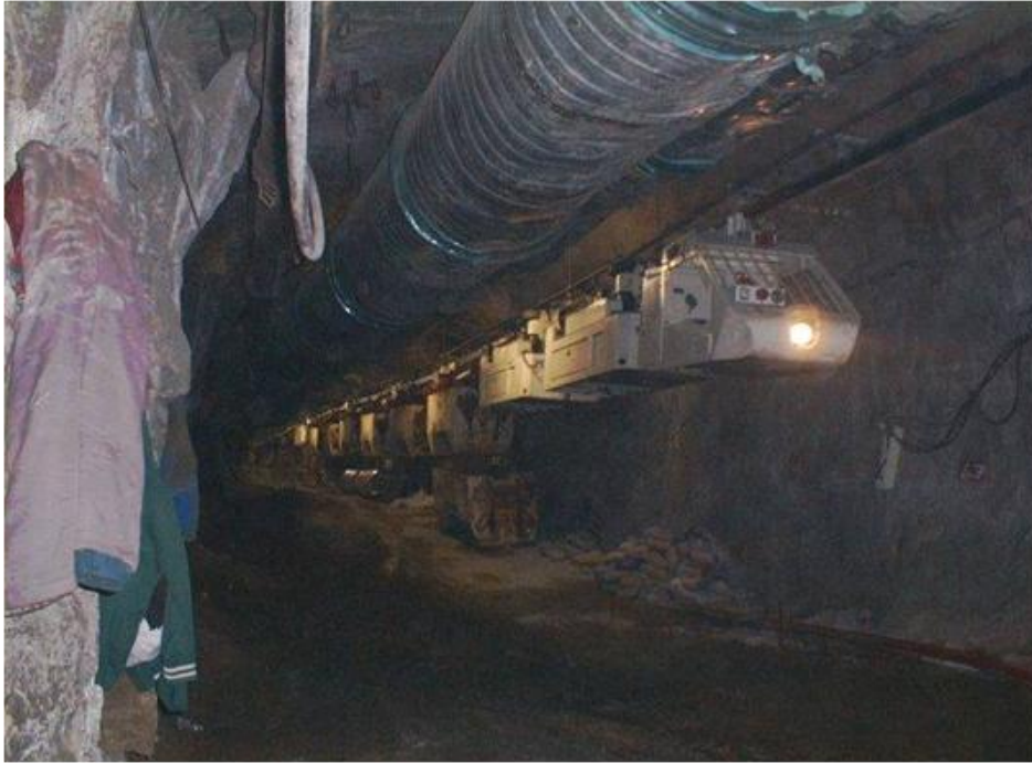
Figure 2.2: EMTS in an underground haulage (Scharf, 2007)
