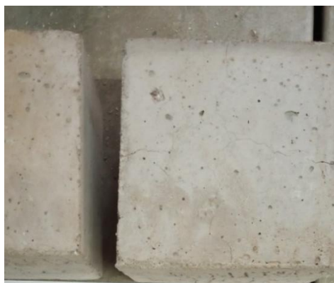
Figure 4.44: Cracks and minor pitting on 10% LCA concrete specimen after exposure to 450°C for 1.5 Hours
