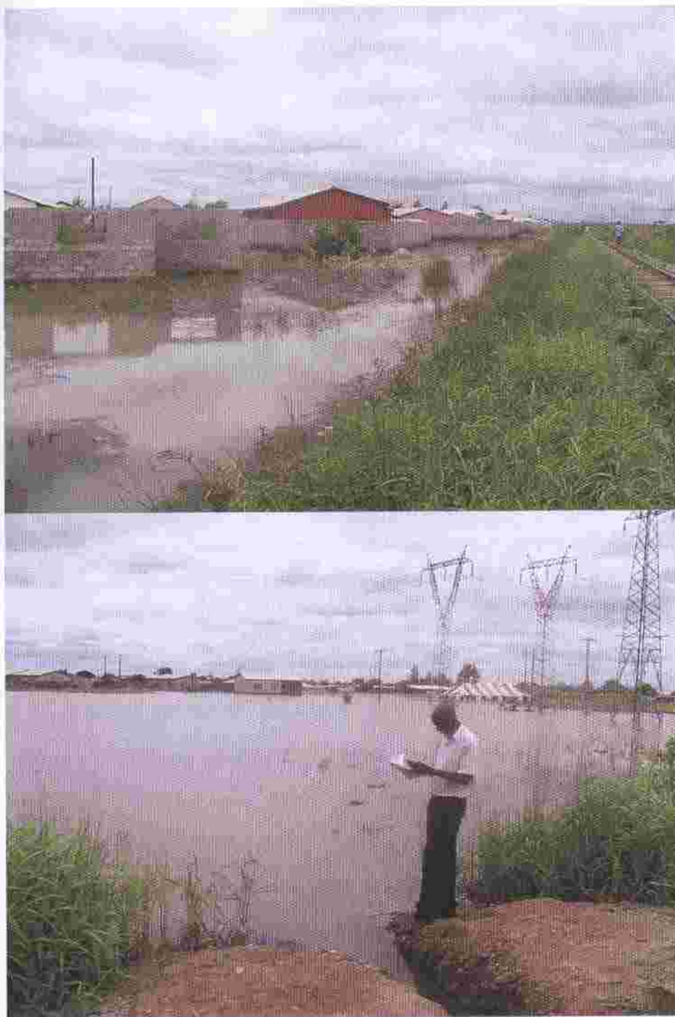
Figure 4.39 Flooding in Kamwala area due to high groundwater table and subsequent accumulation of rain water on Lusaka Plateau: October to December 2007.
