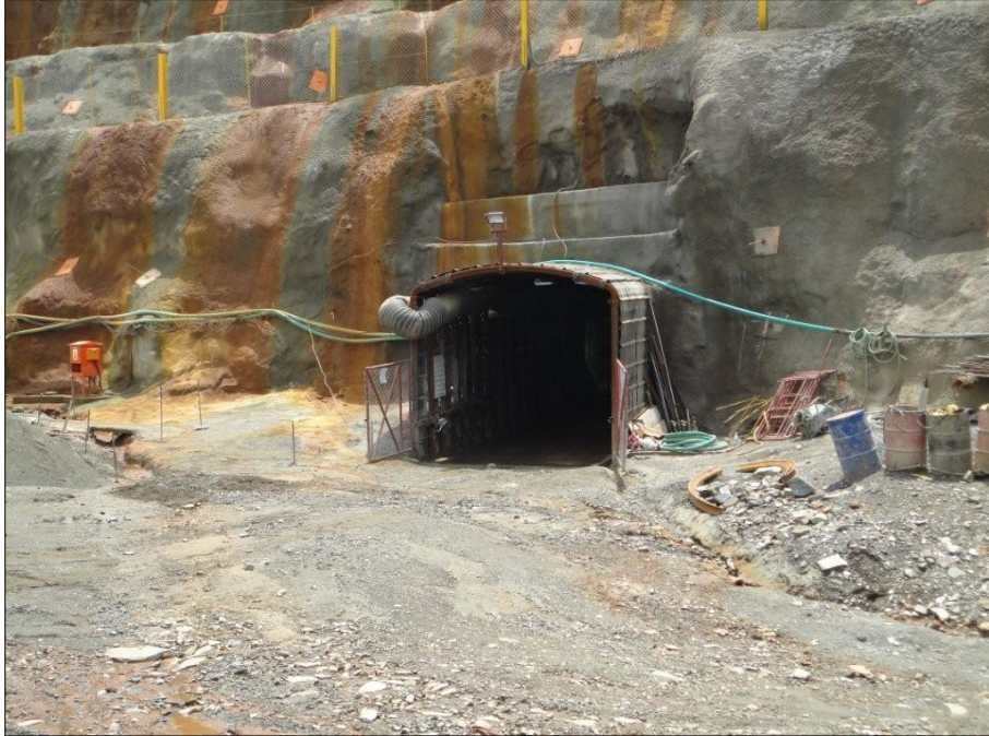
Figure 10 Installed Steel arches at the portal entrance
