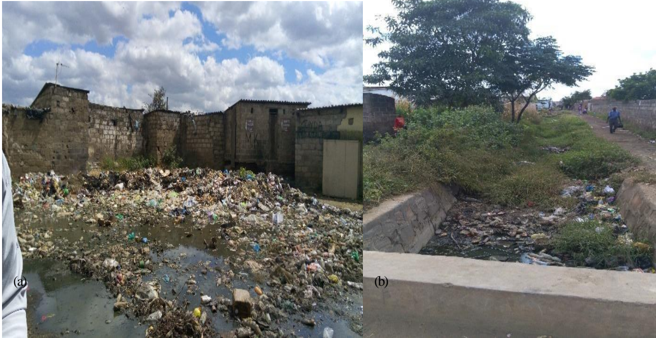
Plate 5.1: (a) Burning /indiscriminate waste disposal and b) Waste disposal in the drainage resulting in blockage of the drainage in Zone 98 of Kanyama Ward 10, Lusaka, 2018.
