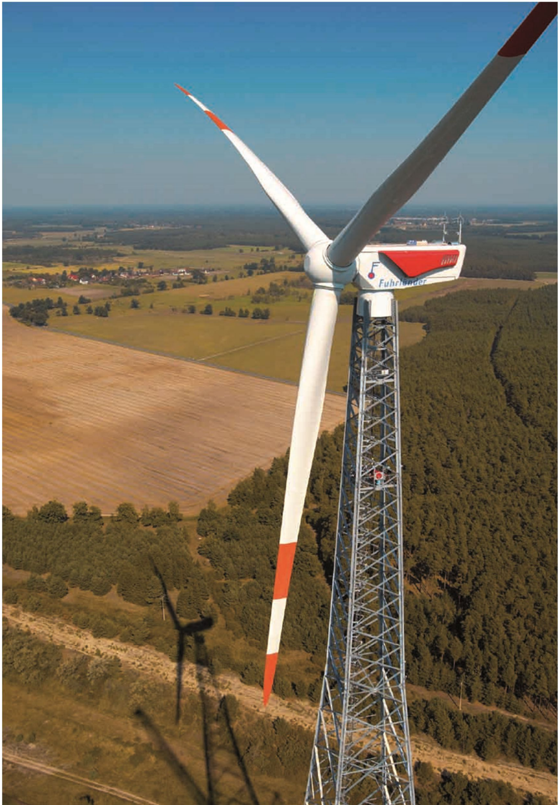
Figure 14: The Fuhrländer Wind Turbine with a 160 m Hub Height Lattice Tower. (Esser-Systems, 2018)
