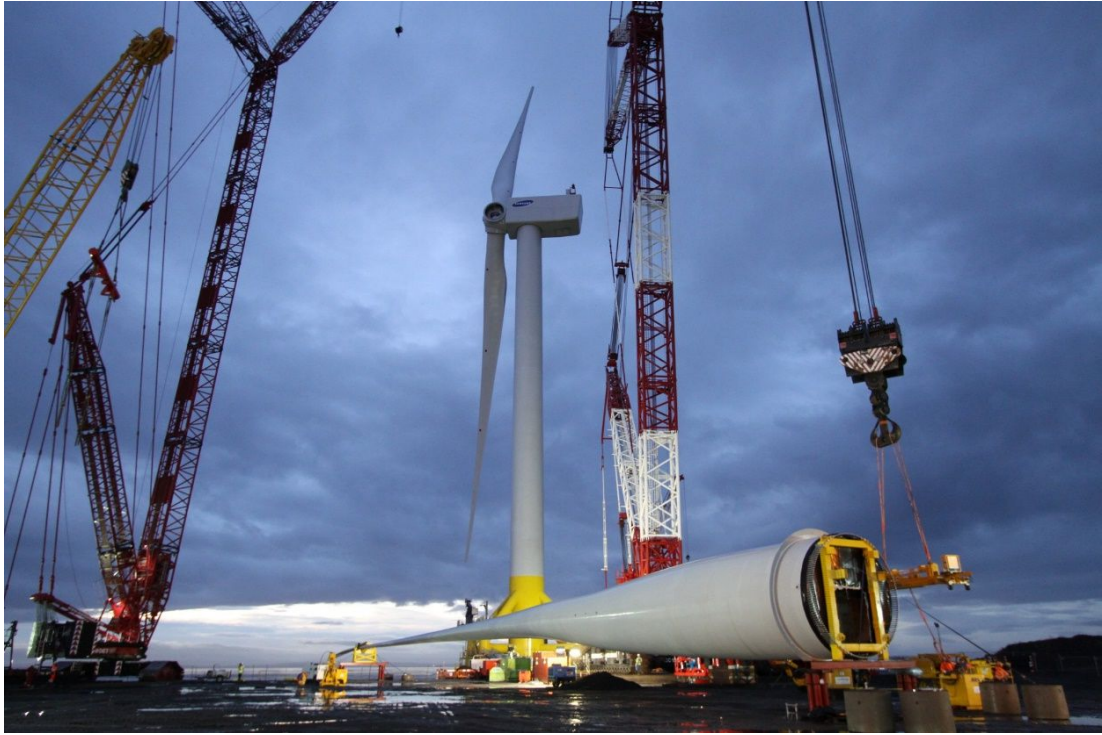
Figure 19: Wind Turbine Installation ( SSP-Technology, 2017 )
