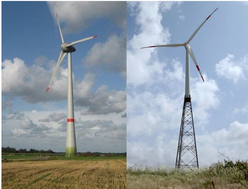
Figure 16: WTs with Hybrid Concrete-Steel Tower and Lattice-Steel Tower.
