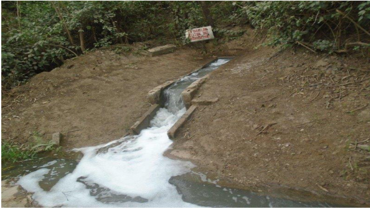
Figure 3.3 Toe drain discharging water.
