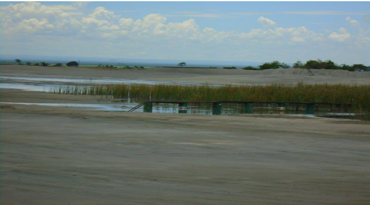
Figure 3.2: Tailings dam walls.
