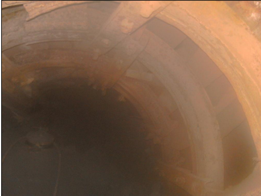
Figure 4.8: Steel set support (Photo: 2420 6E 7B scraper drift)
