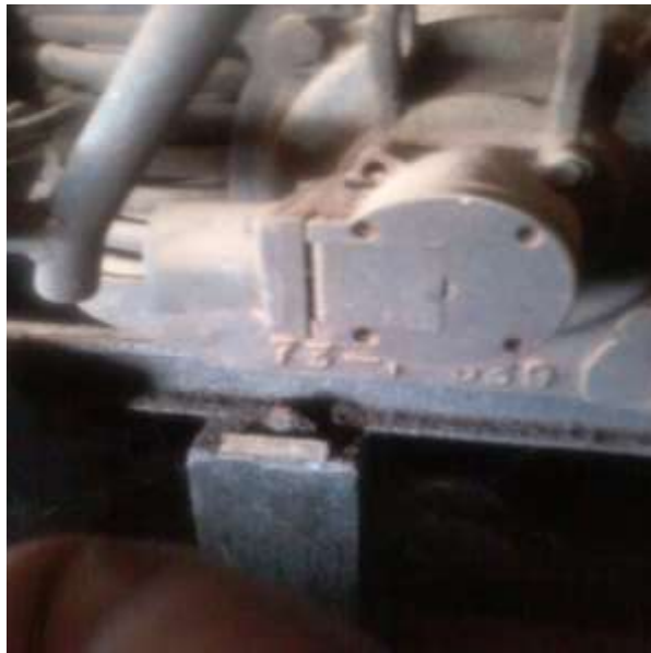
Figure 1.3: Unshielded DFH 2 transducer connected to the wheel axle.
