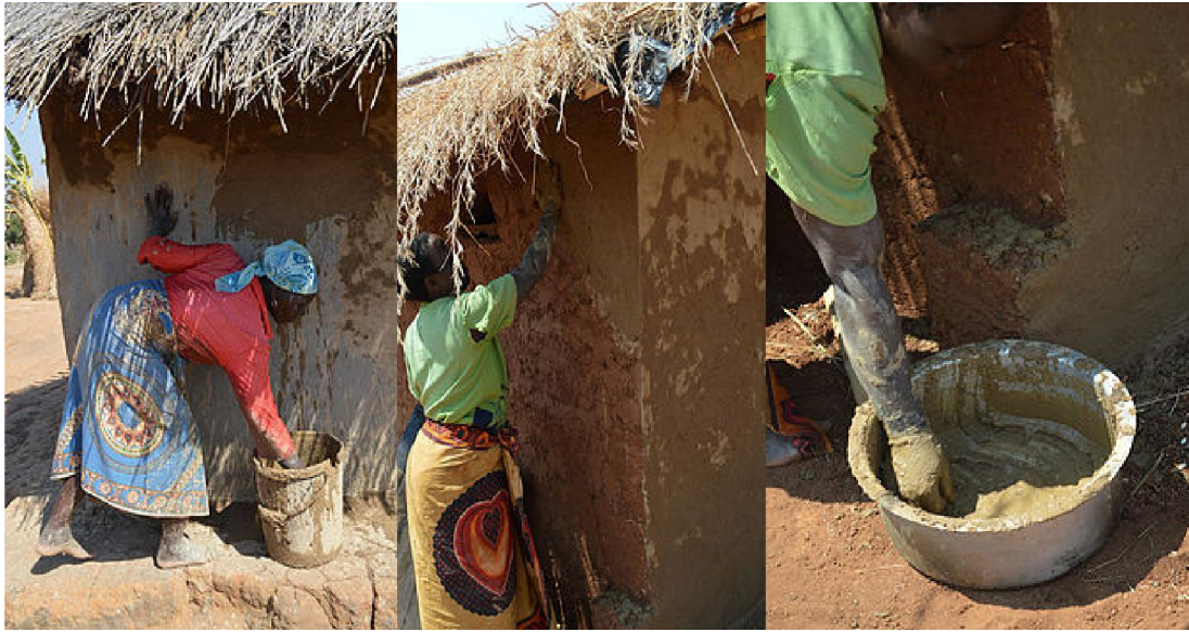
Figure 2.9 Plastering the houses – (Malawi Vernacular Architecture 2011)
