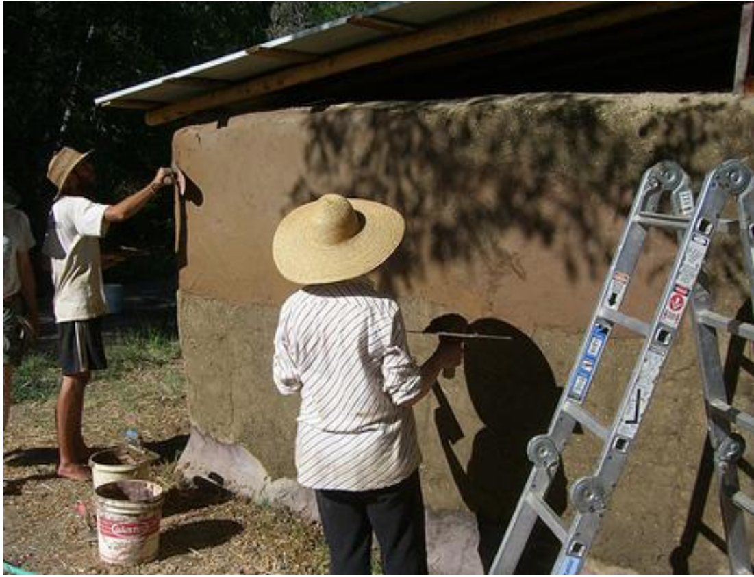
Figure 2.4 Application of earthen plaster – (Photo Source: Ziggy 2008)
