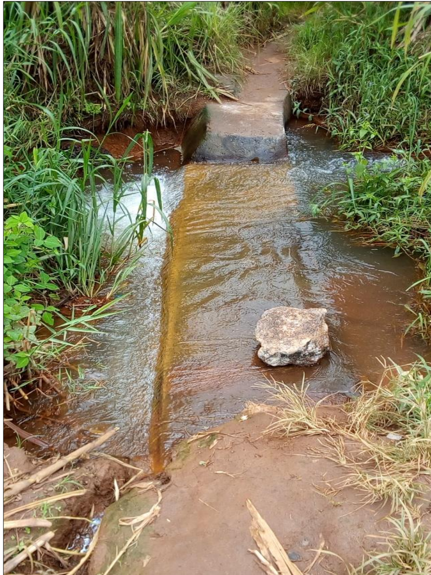
Figure 3.2: The weir on the Chiweta River for Kamgultse irrigation scheme
