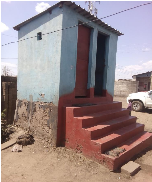
Figure 22: Raised Latrine in Kanyama
