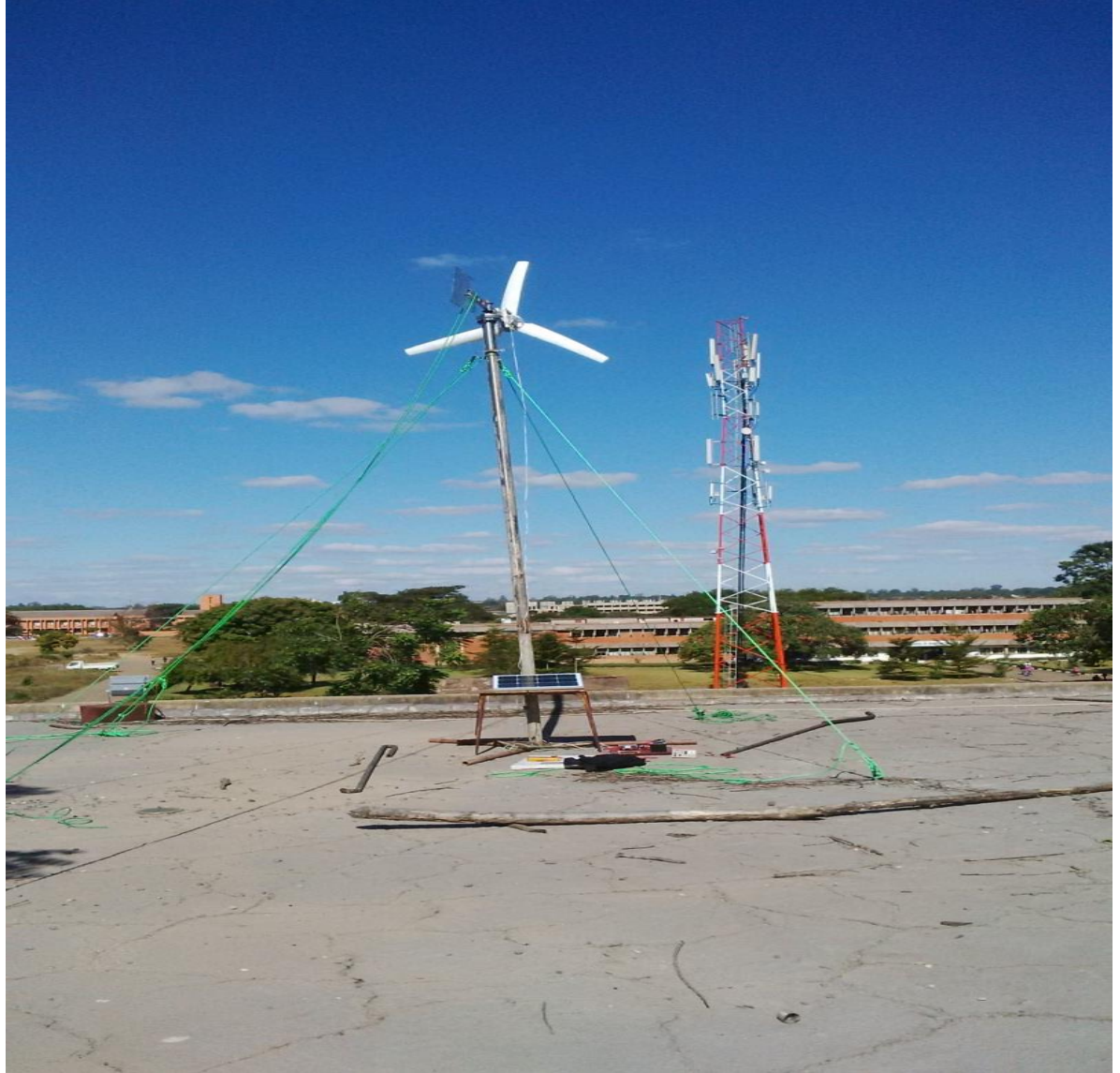
Figure A2.4: The Hybrid in action at the School of Engineering.
