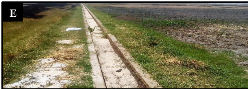
Figure 41: Photographic evidence of sedimentation yield in river channels and the main Barotse Floodplain: (A) and (B) main irrigation canal showing sediment accumulation, (C), (D) and (E) shows sedimentation in the branch irrigation canals and (F) shows sedimentation in the main Barotse Floodplain on the banks of the Zambezi River, Western Zambia.
