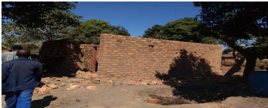
Figure 4. 30: A new house being constructed
