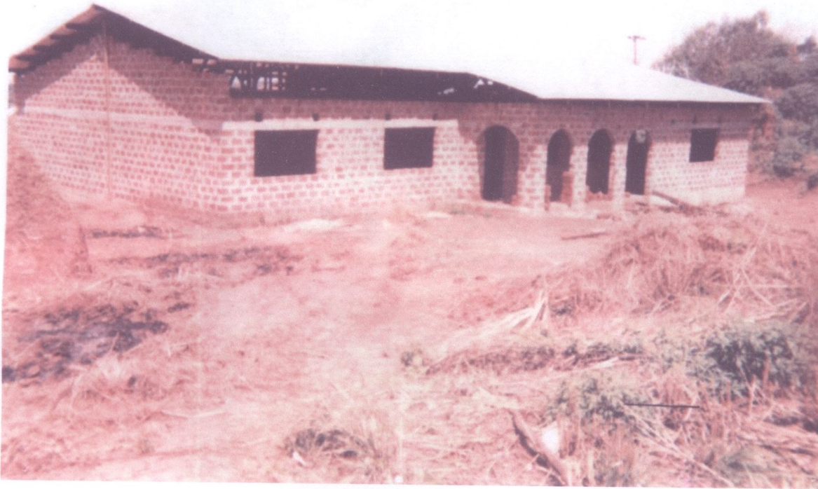
Plate 3: Misplaced high-cost housing in front of ZAWA offices in Solwezi urban, 2005
