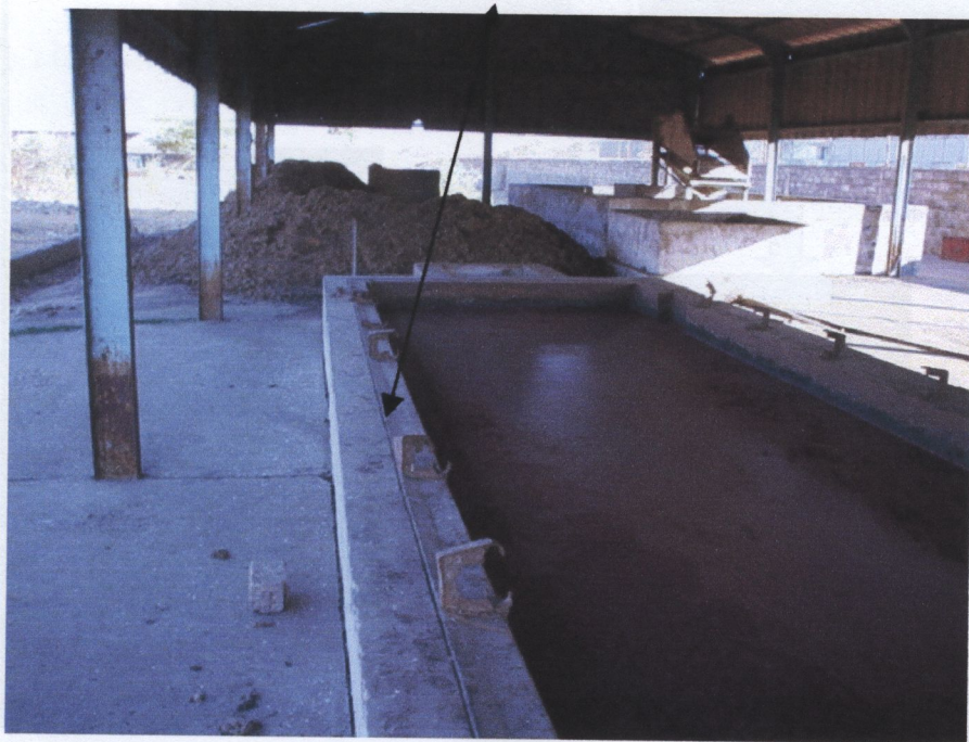
Manure pit-recharge tank
