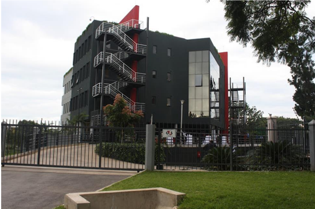
Figure 4.1-11 Exterior View of Citibank Head office
