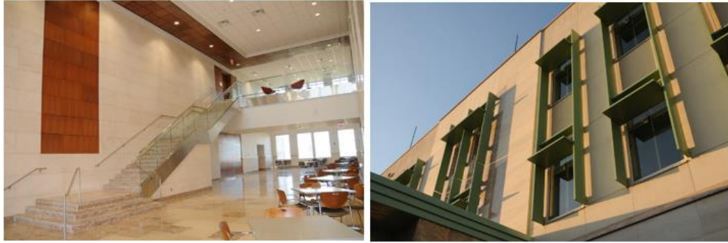
Figure 4.1-13 Natural lit hall and shading devices on exterior
