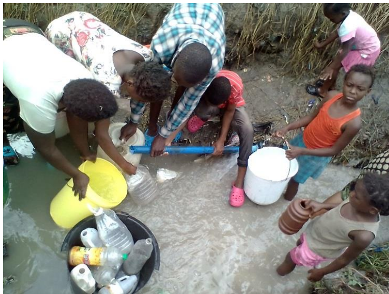
Figure 7: Residents draw water from a vandalized pipe
