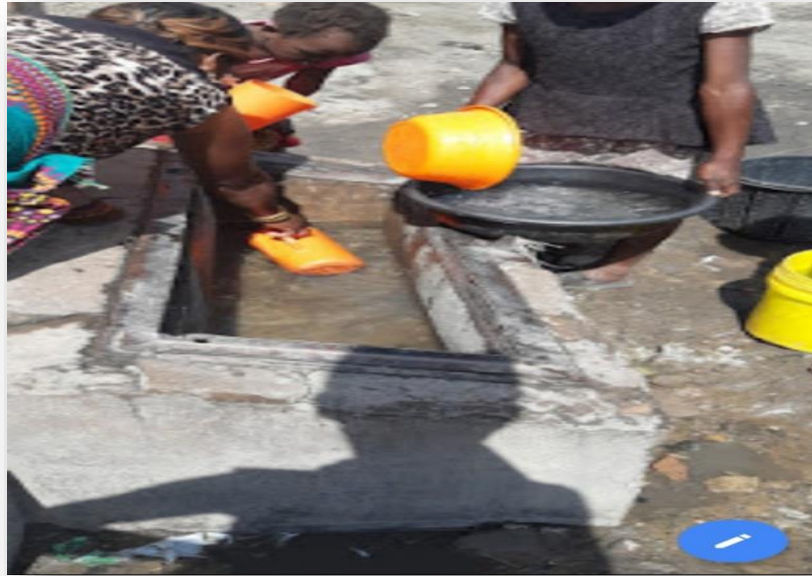
Figure 5: Women and girls tap water from a broken pipe at the kiosk Source: Field data, 2019
